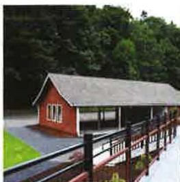
BEACH PARK PICNIC SHELTER
